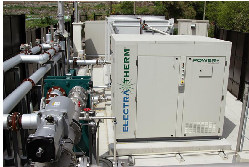
ElectraTherm unit installed in Japan on an onsen geothermal resource
