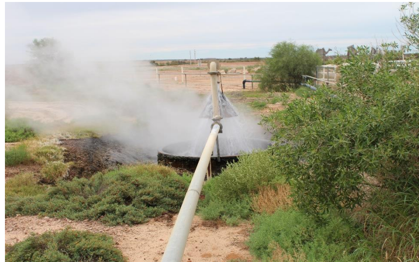
Great Artesian Basin geothermal well (photo : Xatech International)
