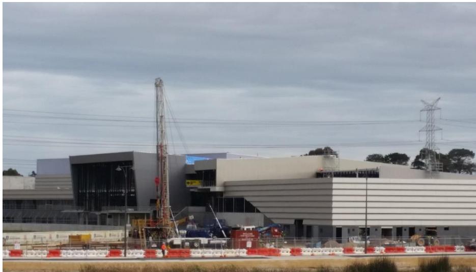
View of the drill site (photo source: Rockwater)
