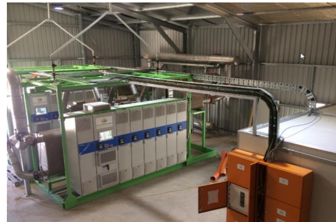
View inside the power station
