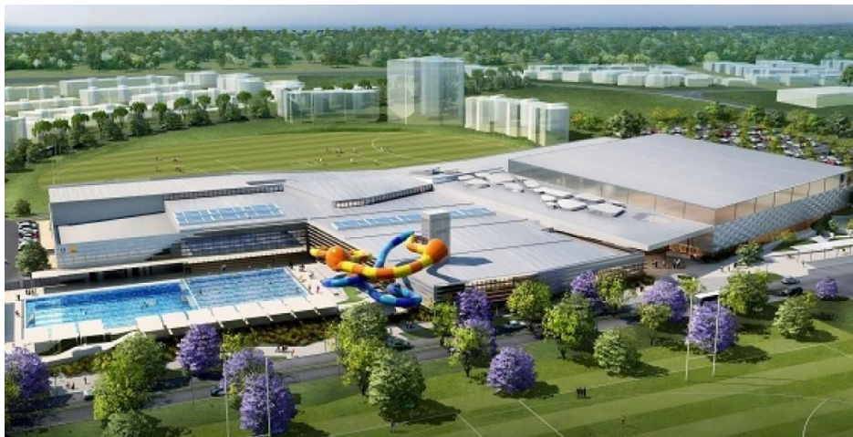
An aerial view of Cockburn ARC, Western Australia, which has a geothermal heating system (photo source: NDY)
