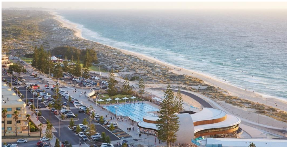
An aerial view of Scarborough Beach Pool, Western Australia, which has a geothermal heating system (photo source: Douglas Mark Black Photography)
