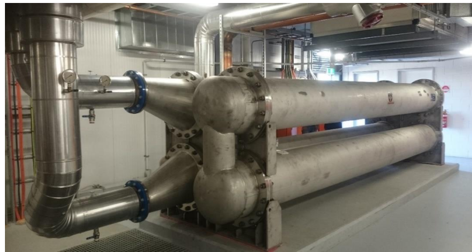
Tube heat exchanger used to cool the supercomputer (photo source: Rockwater)
