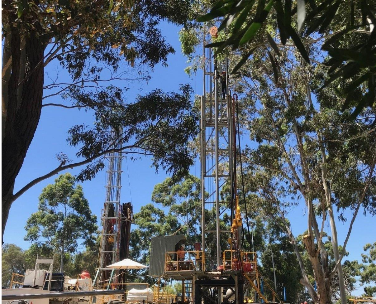
View of the drill site (photo source: Rockwater)
