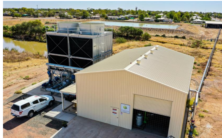
An aerial view entire power station
